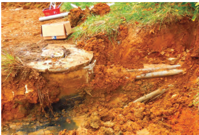
The EPA made several revisions to the 1988 UST regulation and the 1988 state program approval (SPA) regulation to help ensure all USTs in the United States meet the same release protection standards.
